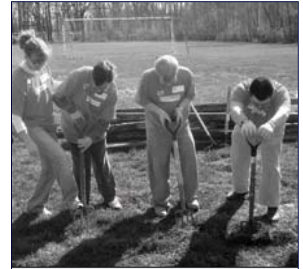
Home Depot and Ken's Krew volunteers prepare to dig a new walkway that leads to the greenhouse.
